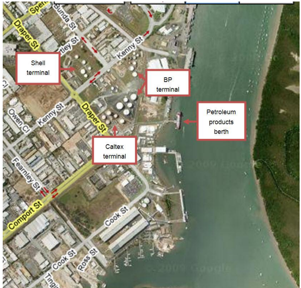
Figure 29 Cairns petroleum product terminals and berth
