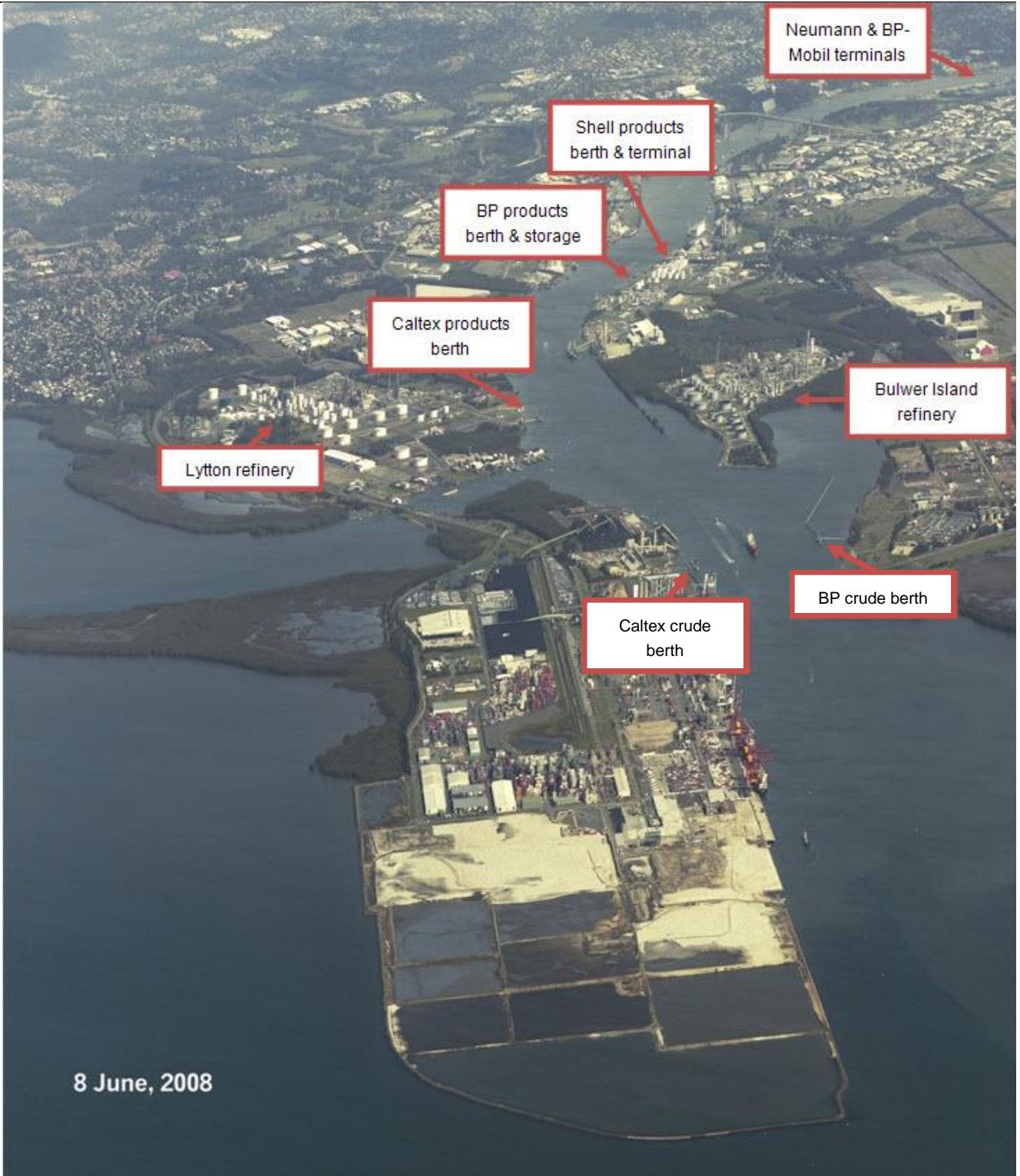
Figure 22 Port of Brisbane: refineries, petroleum berths, petroleum product terminals
