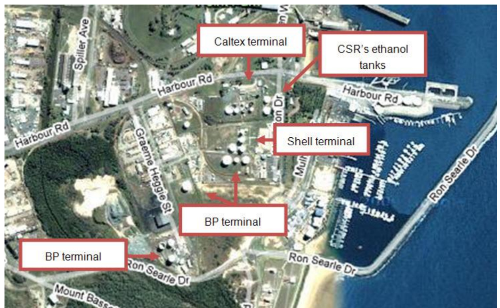
Figure 25 Port of Mackay and petroleum products berth and terminals
